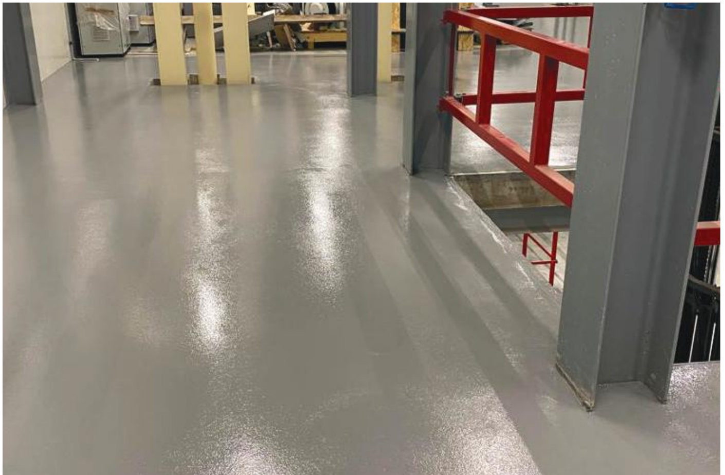
Texture 2 was installed to provide the right anti slip
